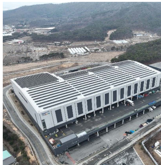
Roof-style solar power plant in Icheon City
