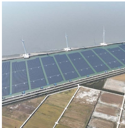
Floating solar power plant in Yeonggwang-gun
