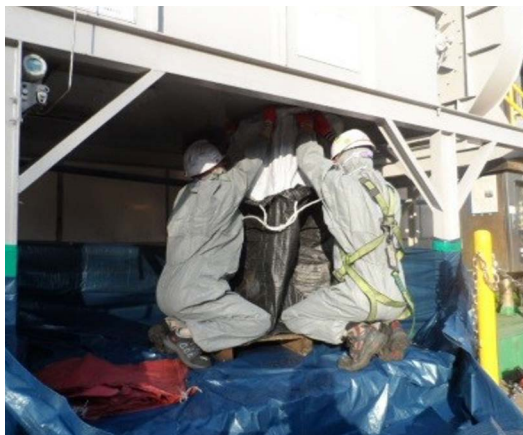
Replacement of adsorption tower activated carbon (1 st and 2 nd half)
