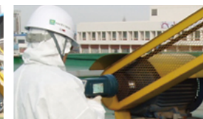
Prevention facility inspection
